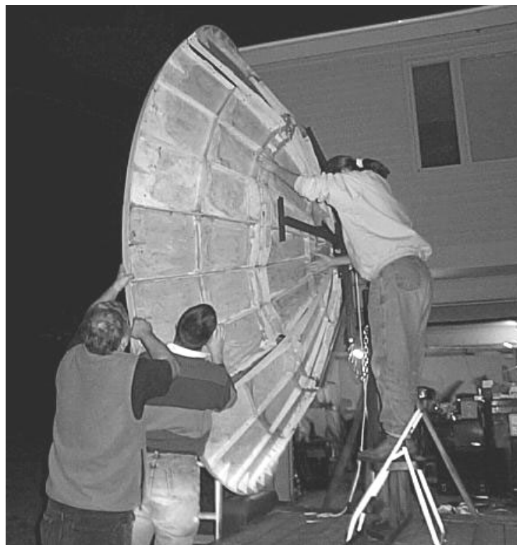
Figure 16: Wedging the third quadrant into place
