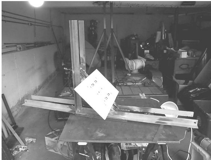
Figure 7: Mounting bracket between dish and elevation mounting plate. (The elevation mounting plate is the white plate in the center of the photograph. The counterweight rails were later welded on as extensions of the vertical bars.)
